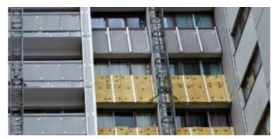
**External thermal insulation 30%** heating savings Gain of up to **3** energy classes
